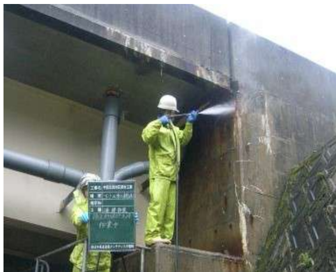
桁端部塩分洗浄状況
