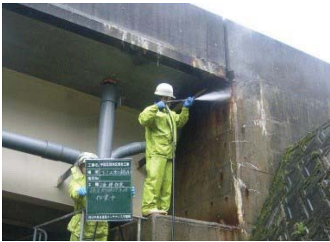
桁端部塩分洗浄状況
